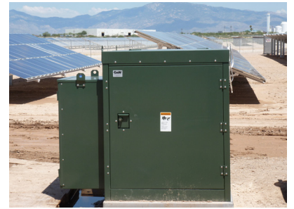
Padmounted Viper-S recloser used in place of a circuit breaker in a solar generation intertie application
