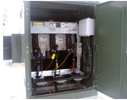
Padmounted Viper-S recloser used in place of a circuit breaker in a solar generation intertie application
