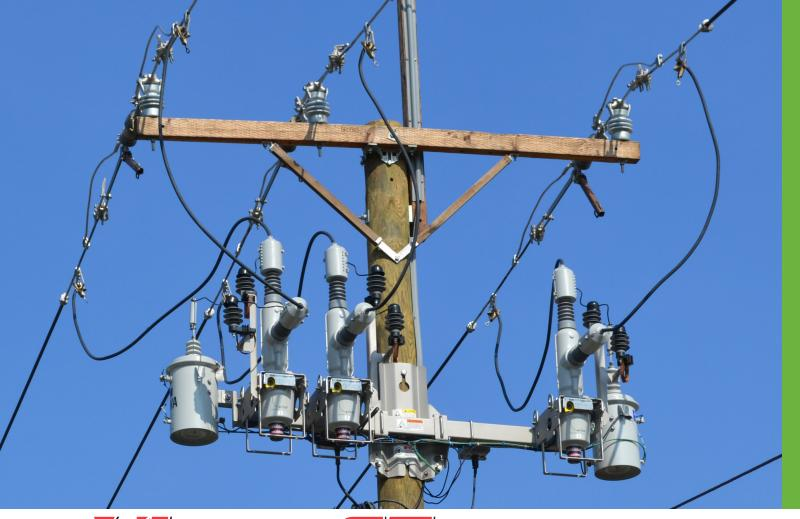
Solid-Dielectric, Independent Pole Option Recloser Providing electronic overcurrent protection for single or three phase operation on systems rated through 38kV, 800A continuous current, 12.5kA or 16kA interrupting current
