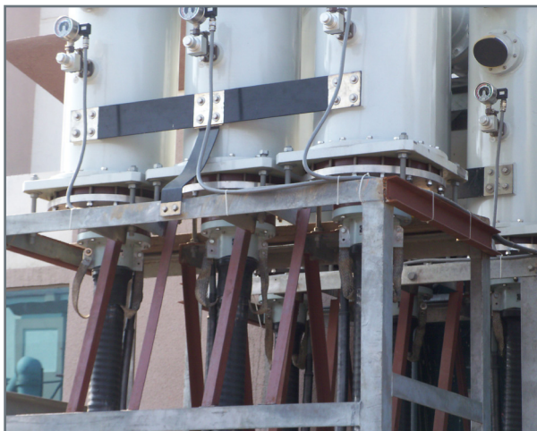
▲ PATR140-SF terminations installed in a GIS.
