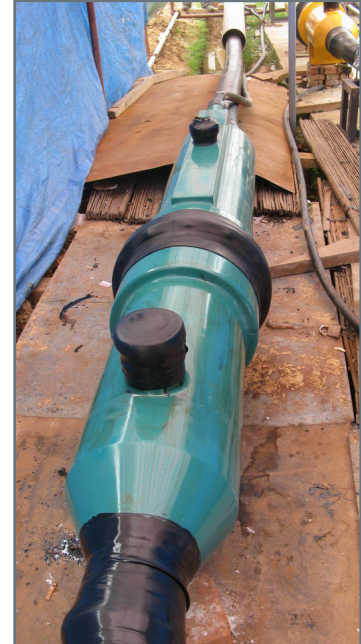
▲ Installation of premolded joint.
