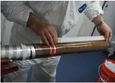
Template for building the stress cone slope is designed per specific cable and provided with the kit.
