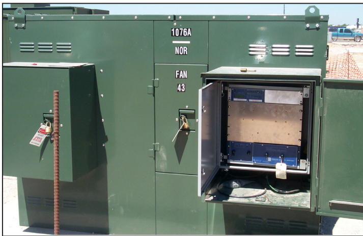
Figure 1: SEL-501-2 control in switch enclosure.
