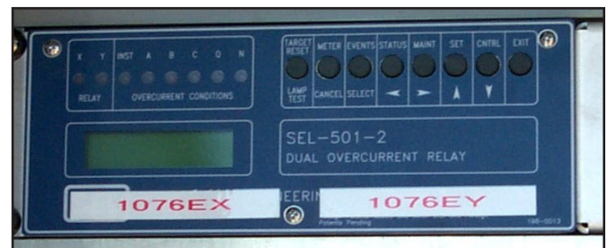
Figure 2: SEL-501-2 control panel close-up
