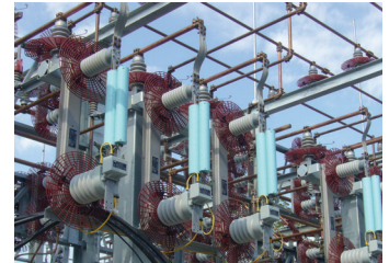
CLiP installed in a generating station at a large southeastern university
